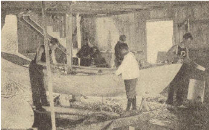
Boat Building at Camp Durrell
